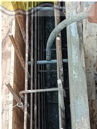
Gambar 4.36 Pengecoran *Shear Wall* 1 (SW.1)
