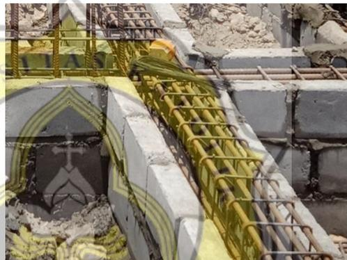
Gambar 3.32 Bekisting *Tie Beam*
