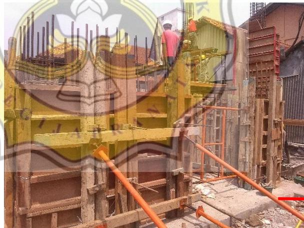
Gambar 4.34 Bekisting *ShearWall* 1 (SW.1)
