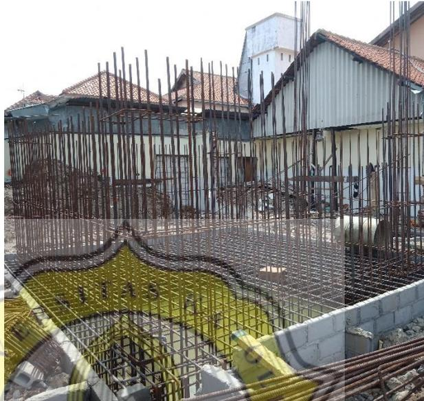
Gambar 4.32 Penulangan *Shear Wall* 1 (SW.1)
