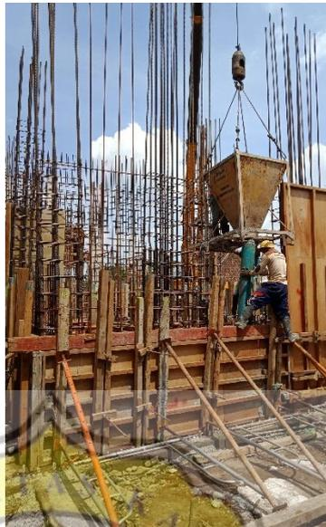
Gambar 4.37 Pengecoran *Shear Wall 3 (SW.3)*
