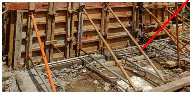
Gambar 4.35 Bekisting *Shear Wall* 3 (SW.3)
