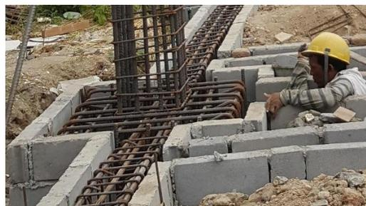
Gambar 3.27 Pemasangan Bekisting *Pile Cap*
