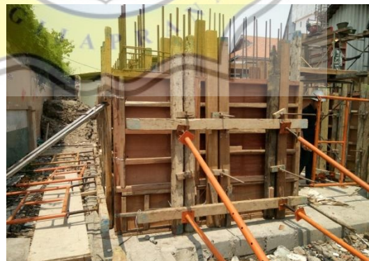
Gambar 3.30 Bekisting Shear Wall Lantai 1
