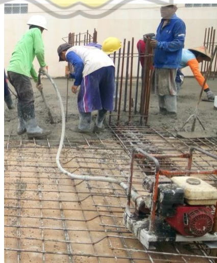
Gambar 3.64 Concrete Vibrator
