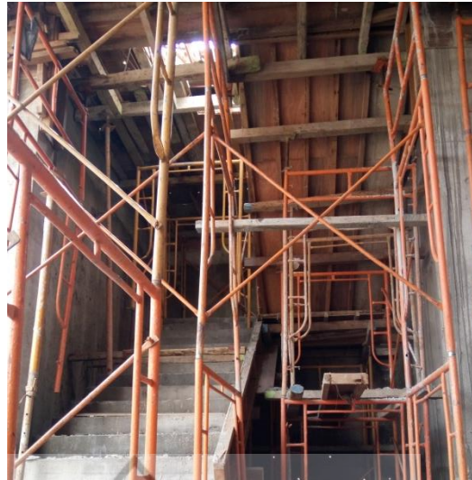
Gambar 3.36 Pelepasan Bekisting Shear Wall
