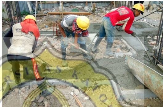
Gambar 3.19 Pengecoran Tie Beam
