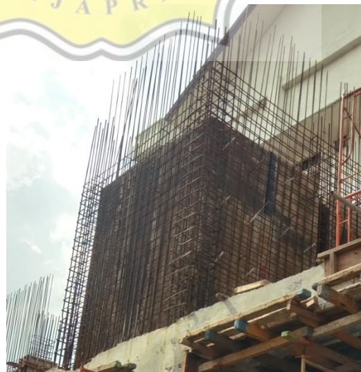
Gambar 3.34 Bekisting Shear Wall Lantai 2
