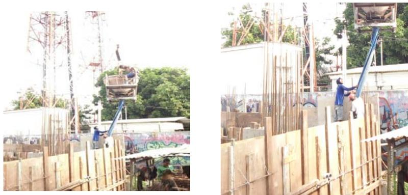
Gambar 3.38 Pengecoran Dinding *Basement*
