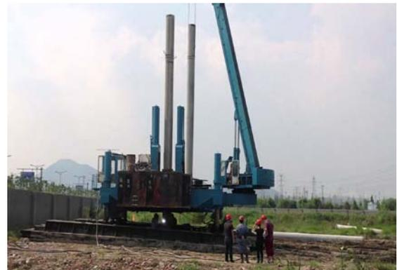
Gambar 3.9 Alat *Hydraulik Static*
