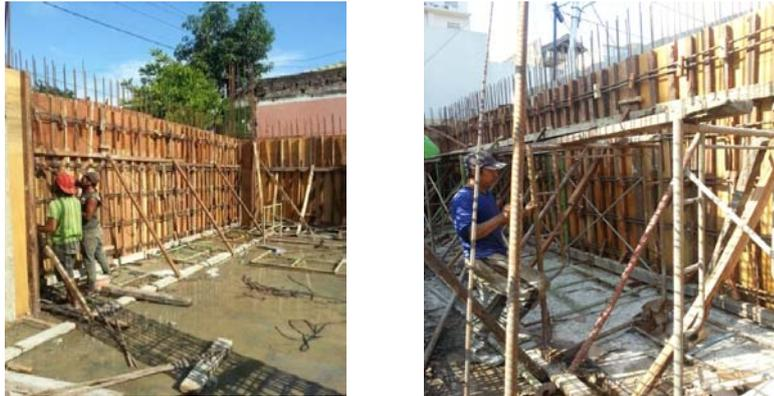
Gambar 3.37 Panel Bekisting Sisi Dalam Dinding *Basement*
