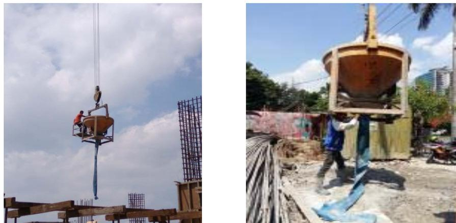
Gambar 3.64 *Concrete Bucket*
