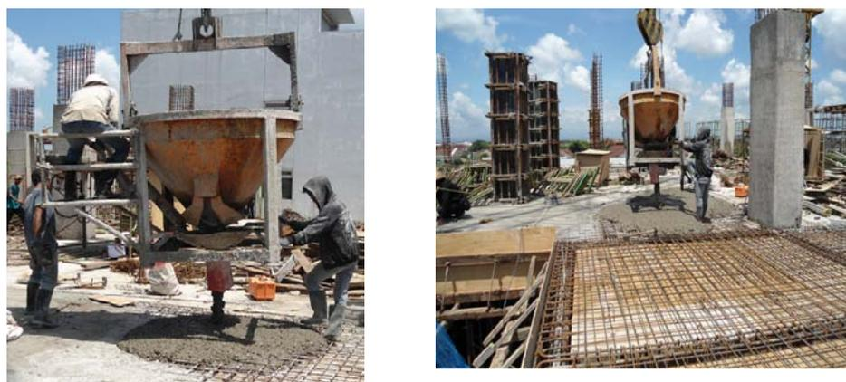
Gambar 3.71 Beton *Ready Mix*
