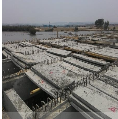
Gambar 3.8 Slab Deck
