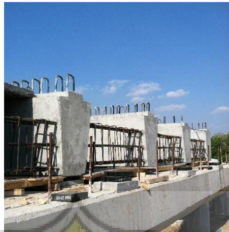
Gambar 3.5 Balok Girder
