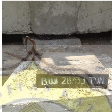
Gambar 3.4 Bearing Pad
