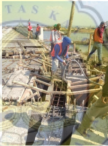
Gambar 3.24 Proses Vibrator
