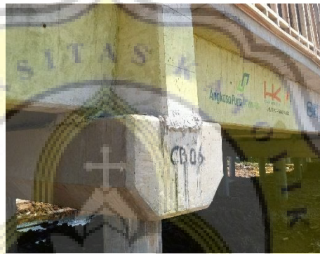
Gambar 3.7 Balok Joint Sendi
