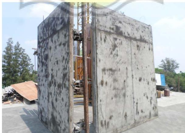
Gambar 3.23 Bekisting Plat *Shearwall*
