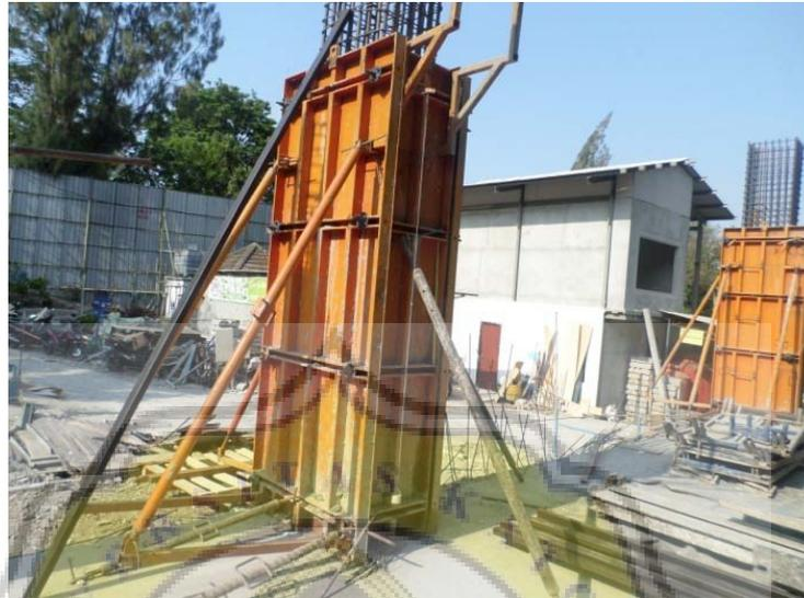
Gambar 3.7 Bekisting Plat Kolom
