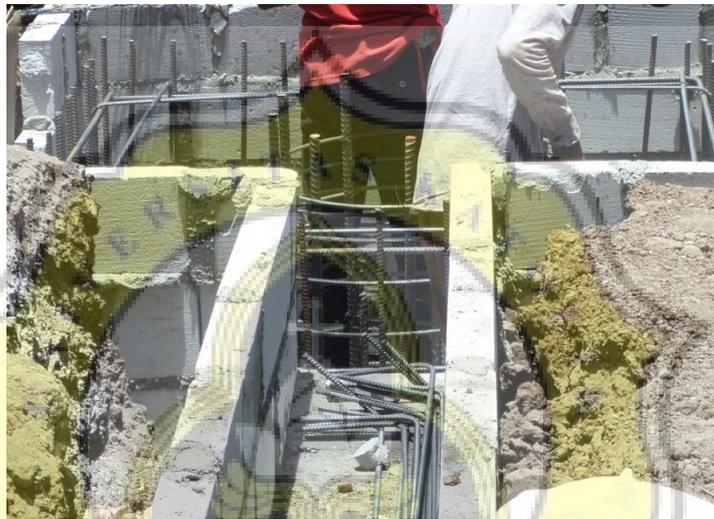
Gambar 3.4 Pemasangan bekisting *Tiebeam*
