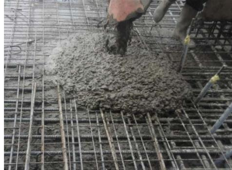
**Gambar 3.72** Beton *Ready Mix*
