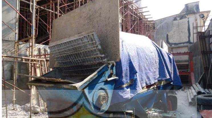
**Gambar 3.66** *Concrete pump* jenis *fixed*
