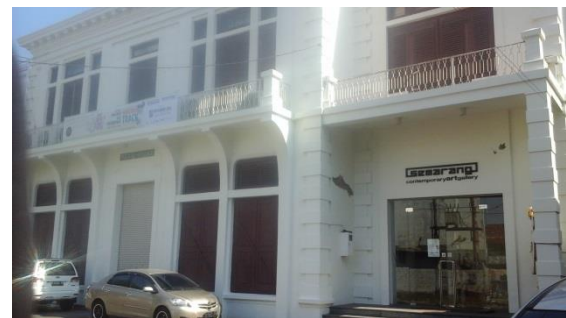
Figure1: Construction activity for building renovation by private sector (2008). This building is a gallery (2014). (Source: survey 2008 and 2014)
