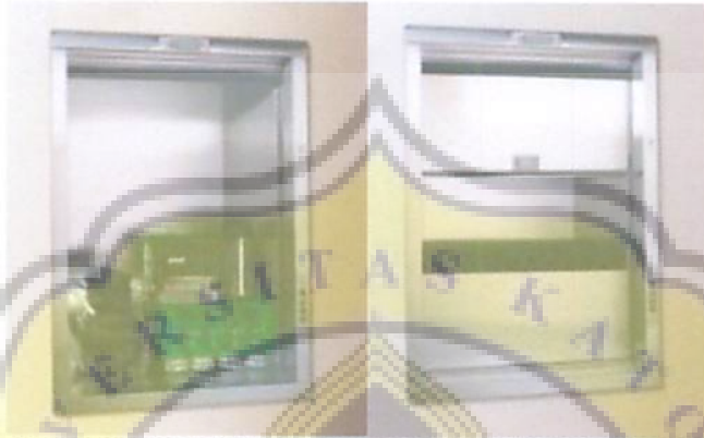
Fig3.23. Dumbwaiter Source : elevatorready.com | January 2013
