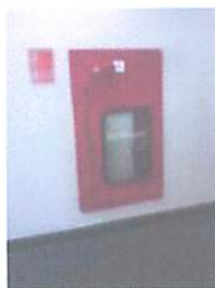
Fig3.30:Hydrant Box
