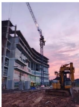
Gambar 3.31 Tower Crane (Sumber: Dokumen PT. SCCR Indonesia)
