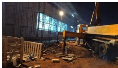
Gambar 4.8 Concrete Pump Truck
