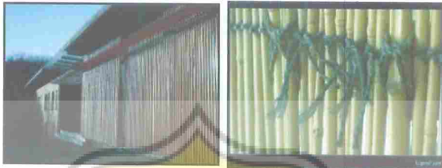
Gambar 4.6 Gambar Lapisan Dinding Bambu
