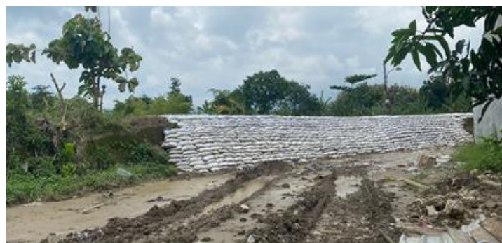
Fig. 1. Emergency Embankment to Replace Damaged Embankment
