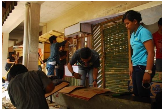
Figure 4: Students building mobile kiosk with recycled and inexpensive renewable building material.
