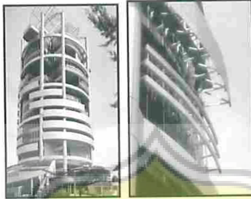
Gb. 5.7 sumber : menara mesiniaga detail architecture enlightens life @ google.com
