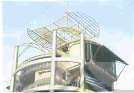
Gb 5.8 sumber : menara mesiniaga detail architecture enlightens life @ google.com
