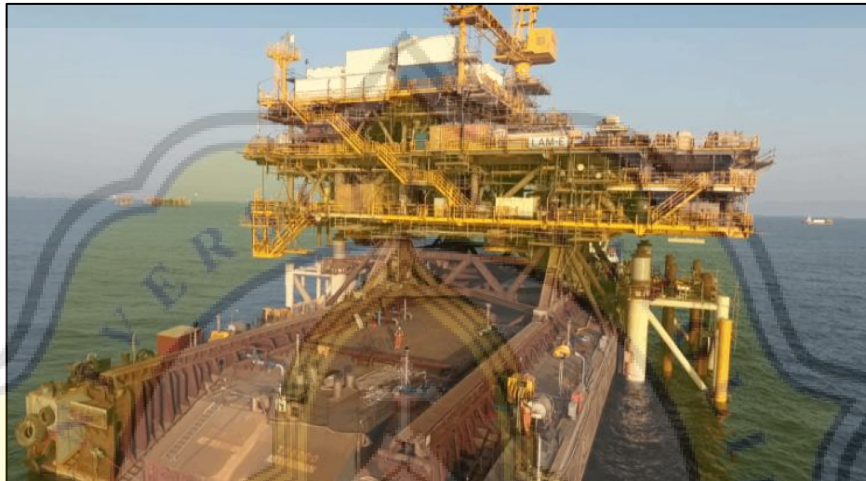
Gambar 4.11. Metode Skidding (Sumber: Pradana, 2015)
