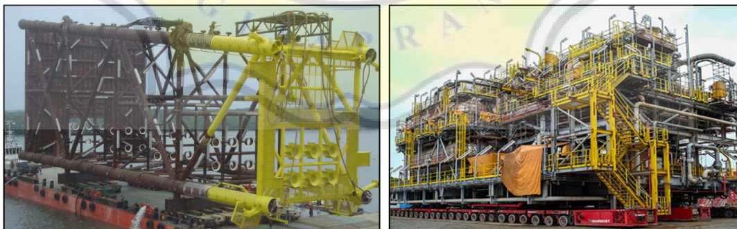
Gambar 4.12. Metode Multi Wheel (Sumber: Pradana, 2015)
