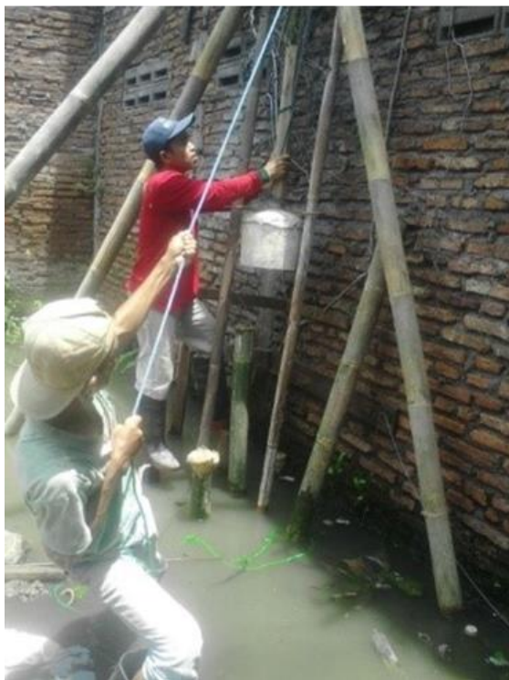
Figure 5: Stacking of bamboo pile at the stage house
