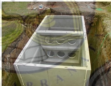
Gambar 56 Konstruksi DWTWC-60000 Sumber : Direct Water Tanks, n.d.
