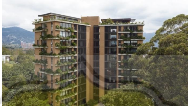
Gambar 32 Avignon Green Building
