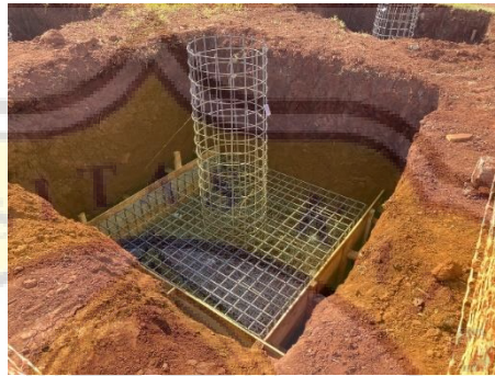
Gambar 6. 18 Pondasi Footplate
