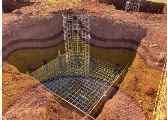
Gambar 3. 21 Pondasi Footplate
