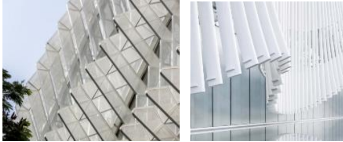
Gambar 106. Perforated Metal Panel dan Aluminium Square Rods Sumber: (Archdaily, 2015)
