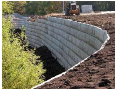
Gambar 219. Retaining Wall (Sumber: https://www.99.co/blog/indonesia/membangun-dinding-penahan-tanah/ )
