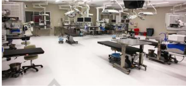
Gambar 230. Monolithic flooring (Sumber: https://www.spectracf.com/lab-flooring/ )
