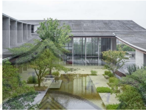
Gambar. Bangunan Utama Yaying Fashion and Arts Centre
