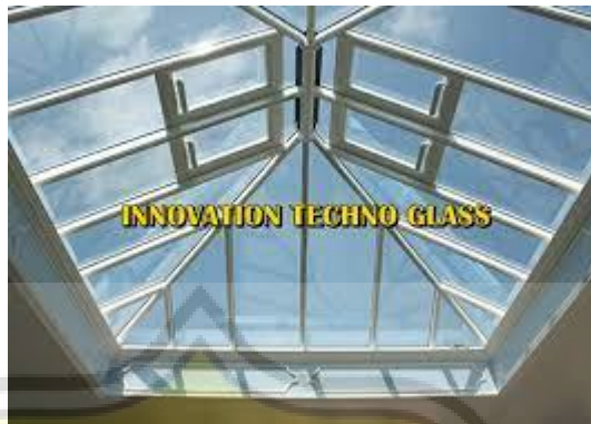
Gambar 6.10 Atap Tempered Glass
