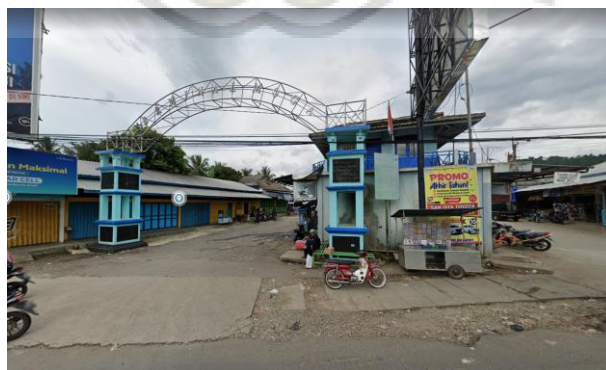
Gambar 34. Terminal Moga (sumber : Google street)
