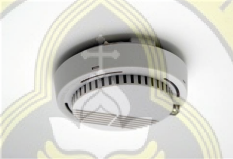
Gambar 63. Smoke Detector
