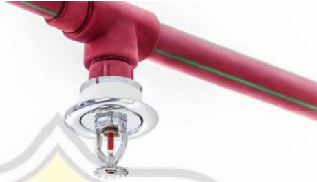
Gambar 6.22. Fire Sprinkler (Sumber : www.google.com )
