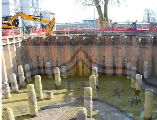
Gambar 24 Pondasi Bored Pile
