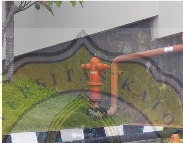
Gambar 4.3.4 Pipa Hydrant
