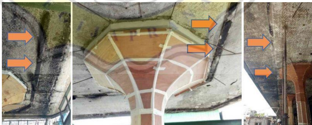
Gambar 4.26. Arang bekas kusen, tersisa angkur lama. Sumber: Sriwati Purnomo, 2017
