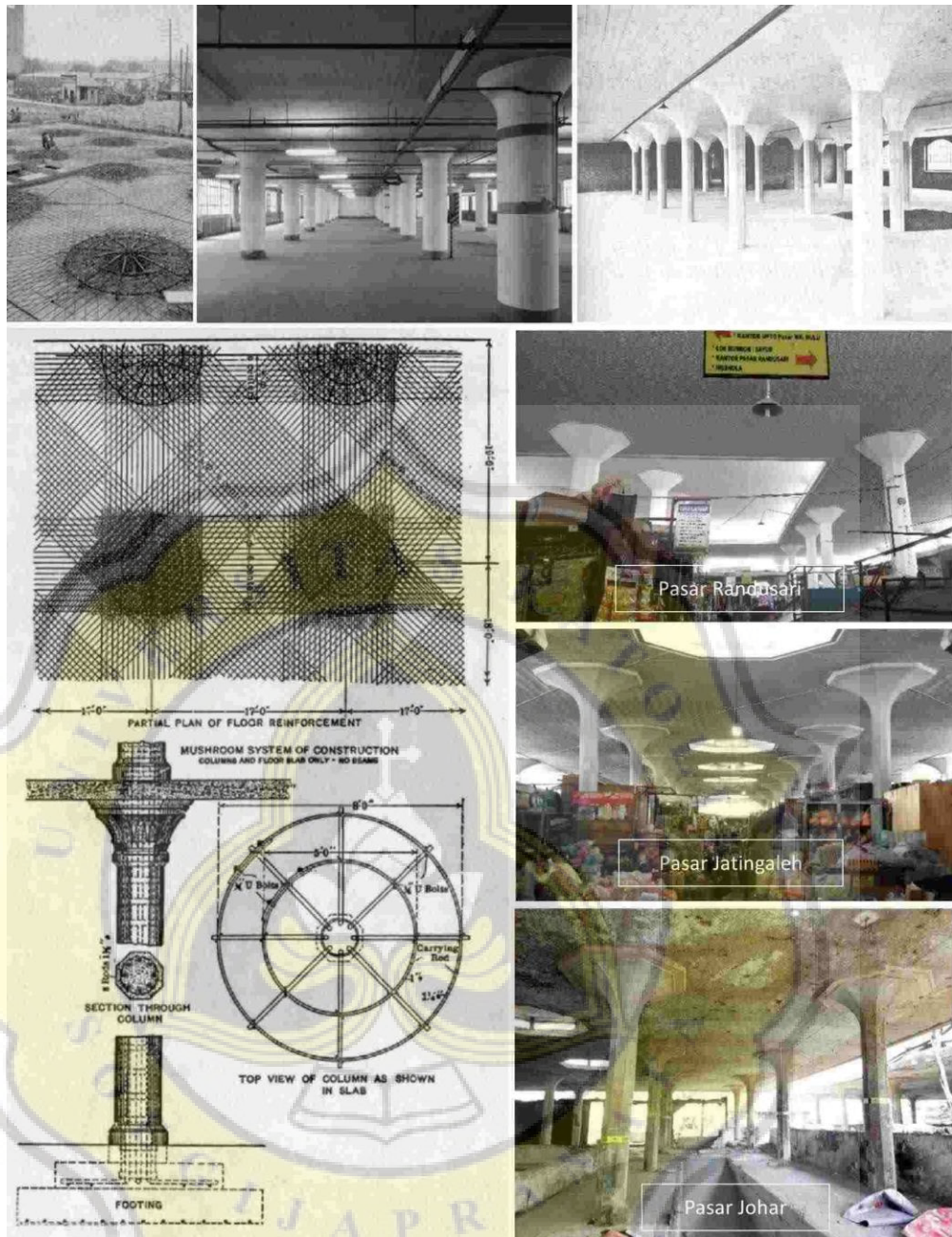
Gambar 4.28. (1,2)C.A.P. Turner: Four-way Flat-plate System, 1909, (3)Robert Maillart: Warehouse, 1910, (4)CAP Turner, details of mushroom slab construction, 1905 (Sumber: Gasparini, 2002, Fig. 6), (5)Tiga pasar karya Karsten di Semarang (Sumber: Sriwati Purnomo, 2018)
