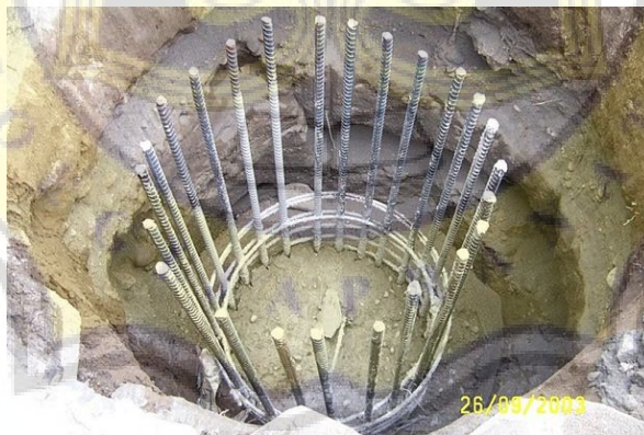
Gambar 3.36 Bored pile
