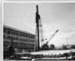
Piles Foundation for Building
