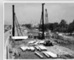
Piles Foundation for Bridges
