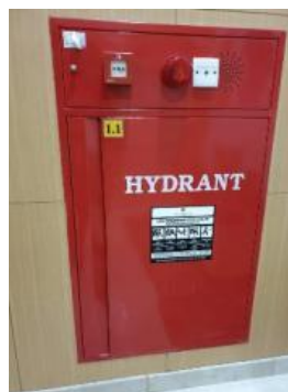
Gambar 7.40 Hydrant Box Sumber : indiamart.com
