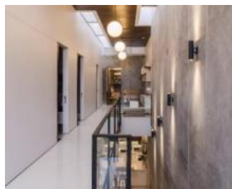
Gambar 7.17 Penerapan Beton Ekspose
