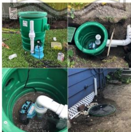
Gambar 7. 36 Sistem Sump pit
