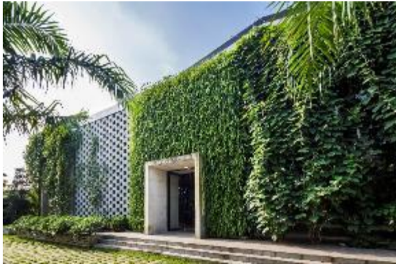
Gambar 69 Fasad DESINO Eco Manufactory Sumber: Archdially.com
