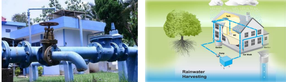
Gambar 7. 8 Utilitas Air PDAM & Rain Water Harvesting
