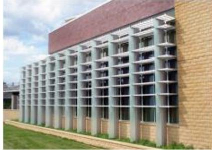
Gambar 39 Egg-crate Sun Shading
