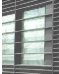
Gambar 37 Horizontal Sun Shading
