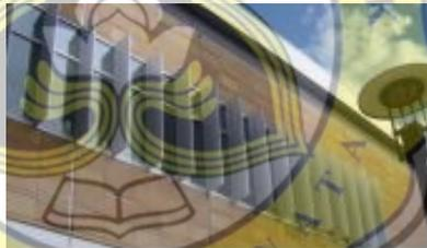
Gambar 38 Vertical Sun Shading
