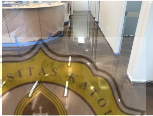
Gambar 68: Lantai Cat Epoxy
