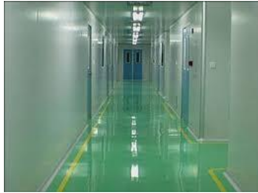
Gambar 87 lantai dilapisi epoxy
