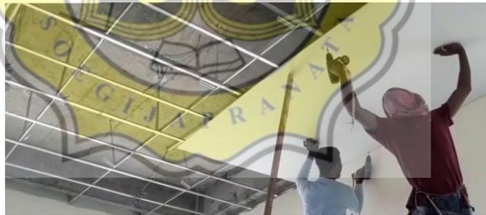
Gambar 33 Pemasangan Gypsum Pada Rangka Langit-Langit(8 Cara Pasang Plafon Gypsum, Pvc, Grc Dengan Rangka Hollow, n.d.)
