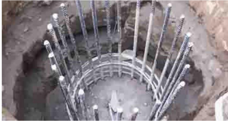
Gambar 18. Pondasi Bored Pile
