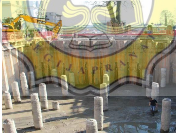
Gambar 37 Pondasi Bored Pile
