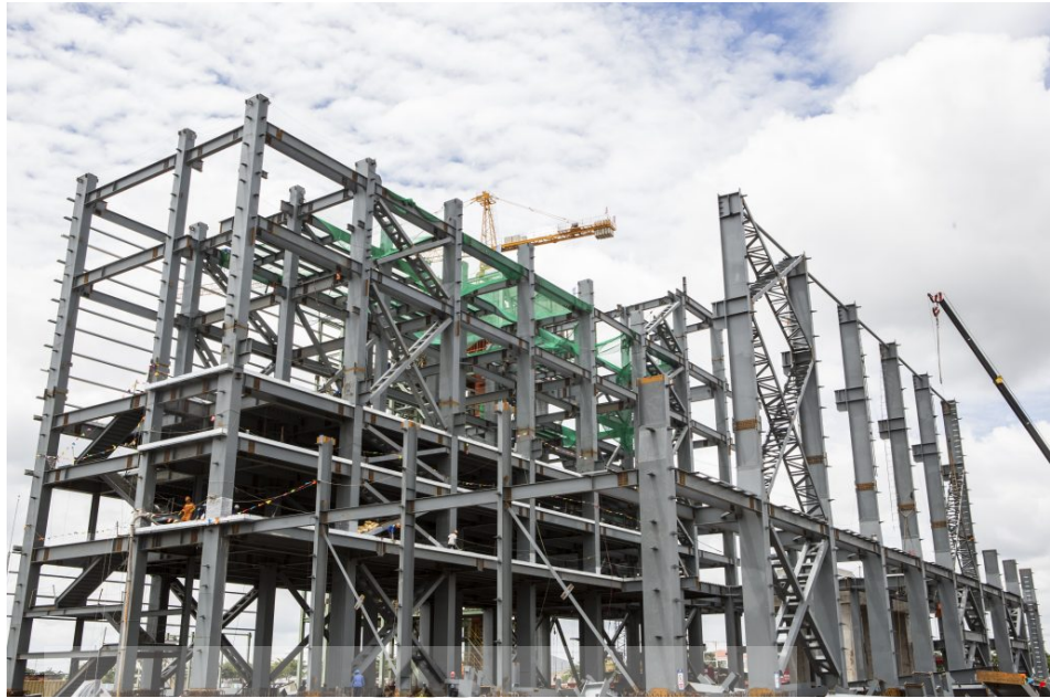
Figure 38. Steel structure (Source: ATAD Steel Structure Corporation)
