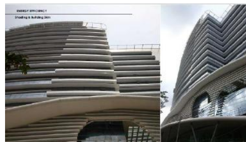
Figure 5. 4 Light Shelves on Ministry of Marine Affairs and Fisheries' Façade
