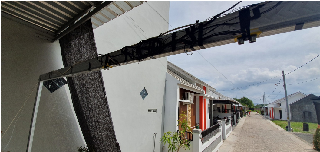
4.2.3 Placement of Ultrasonic Sensors on motorcycle lanes
