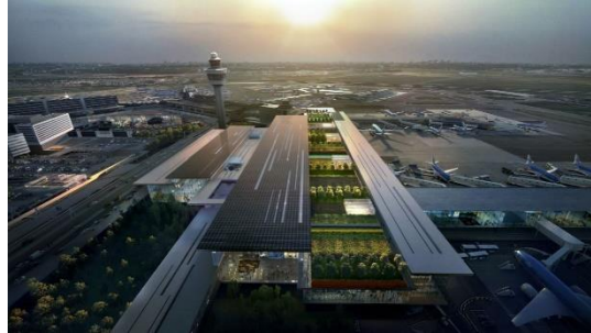
Gambar 83. Roof Top Schiphol Airport Terminal Area A
