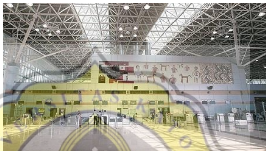
Gambar 7.4 : Airport Spaceframe Structure
