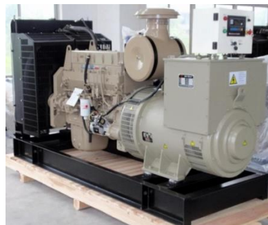
Gambar. 49 Genset Tipe Open Merk Cummins
