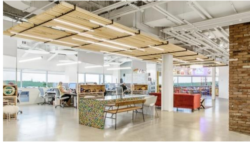
Gambar 33. Ducting AC Central Sumber : google.com
