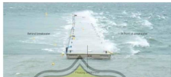
Gambar 88. Floating breakwater (sumber: Floating city)
