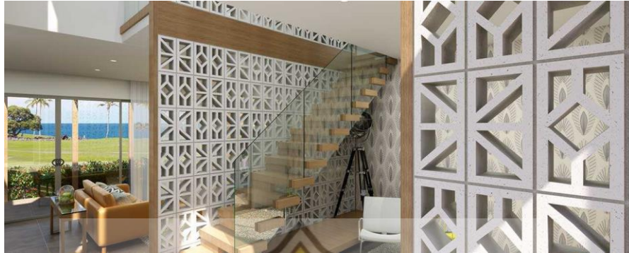
Gambar 39. DINDING ROSTER BETON
